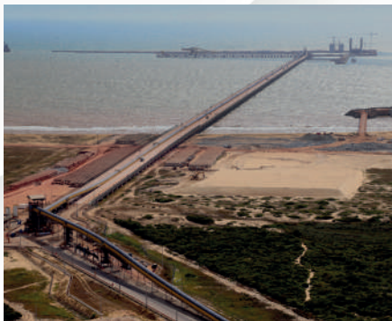
Iron Ore concentrate exportation port - Brazil Overland Conveyor of 3 km High capacity of 20.000 t/h
