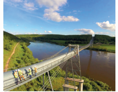
Cement Plant - Russia Overland Conveyor of 6 km Rope bridge to cross a river / 240 m span between pylons
